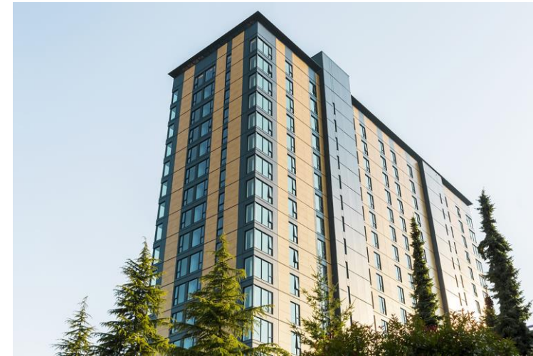
(Tallwood House in Vancouver)
